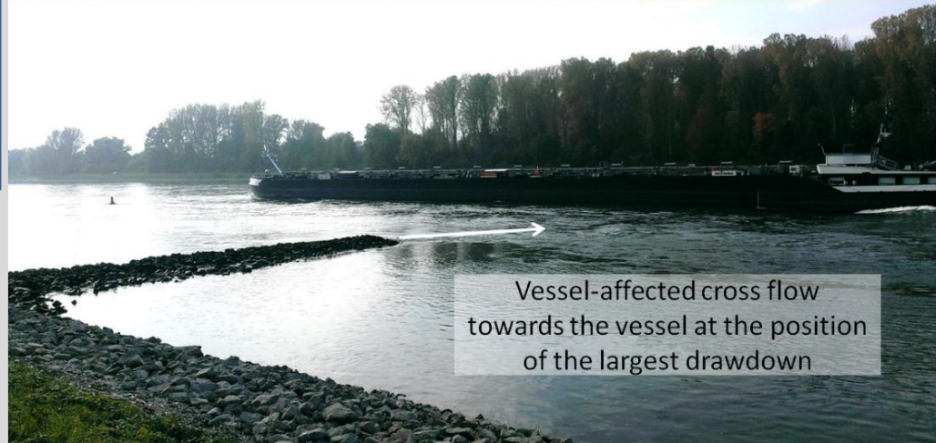
Figure 1: Flow vectors at a groyne head without (upper picture) and with drawdown influence (lower picture)
