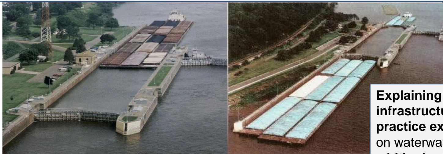
Figure 1: Multiple locking of a pushed convoy in the USA
